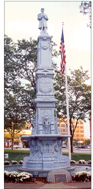
The Kent County monument after its $250,000 restoration.
